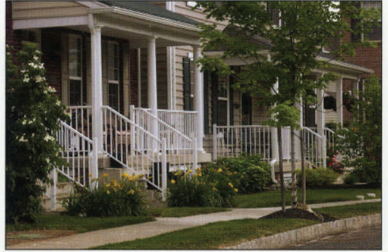
Classic Style Railing at front entrance, townhouse community
