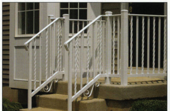
Standard Style Railing with alternating straight and twisted pickets, townhouse community
