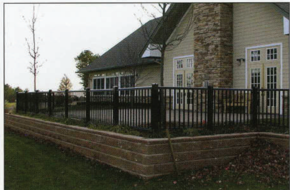
Classic II Style Railing at clubhouse, condominium community
