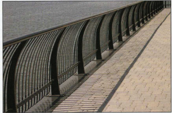
Bowed Fence at waterfront condominiums
