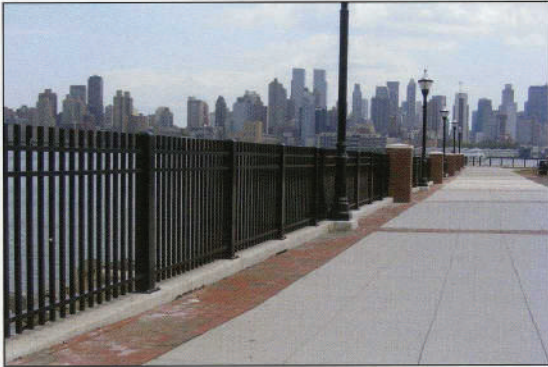
Three Line Picket Fence, community park
